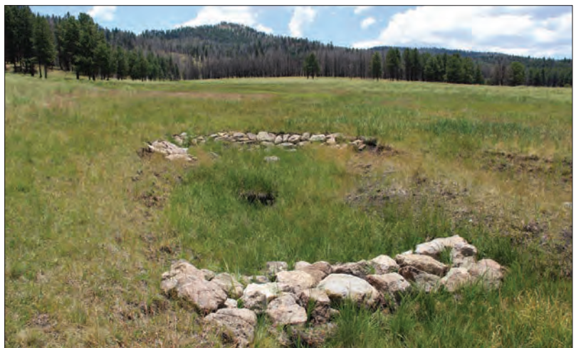
Figure 53. Site 11, July 6, 2017. Paired rock layback and one rock dam as revegetated two years later. (©T.E. Gadzia)
