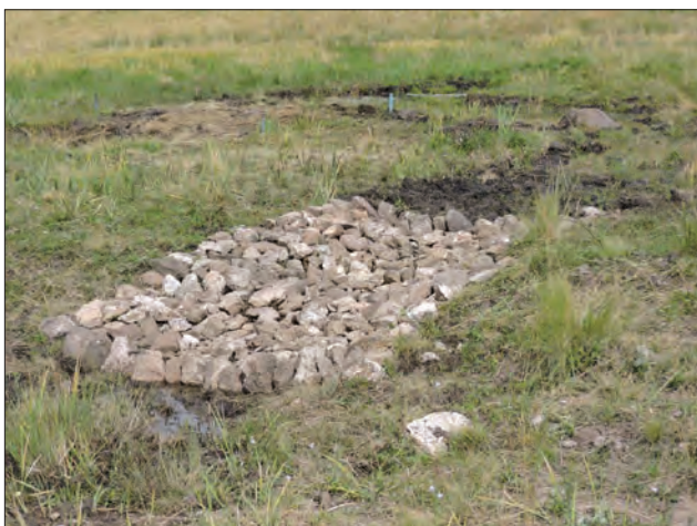
Figure 51. Site 19. Left, rock rundown after construction, August 25, 2015. (©W.D. Zeedyk) Right, two years later, July 6, 2017. (©T.E. Gadzia)
