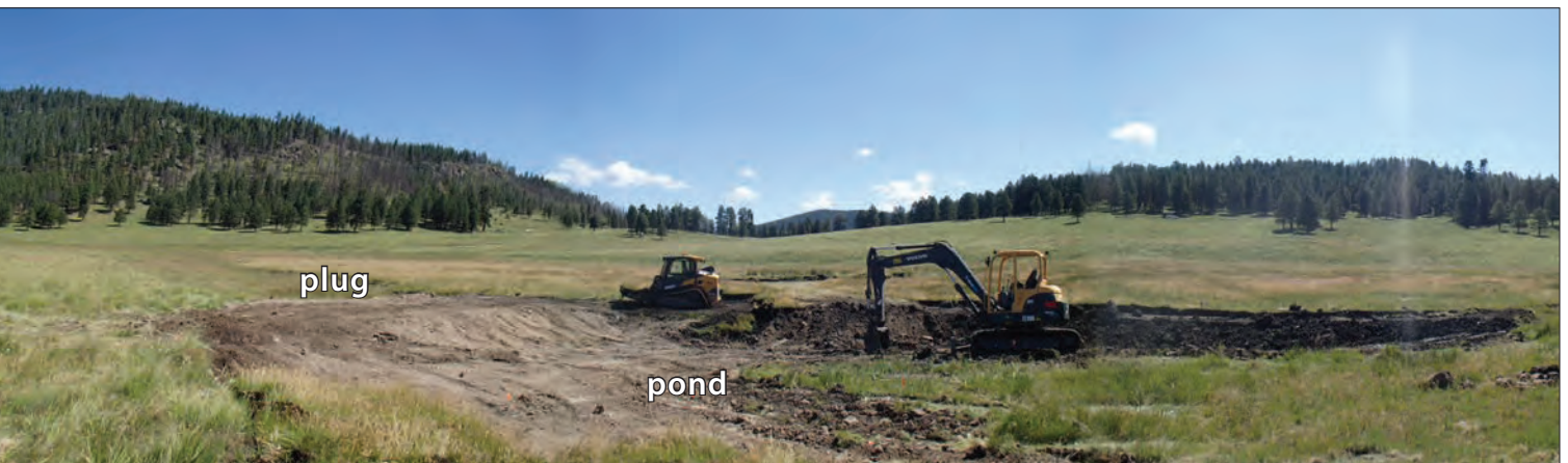
Figure 28. Constructing and compacting the plug. (©S. Vrooman)
