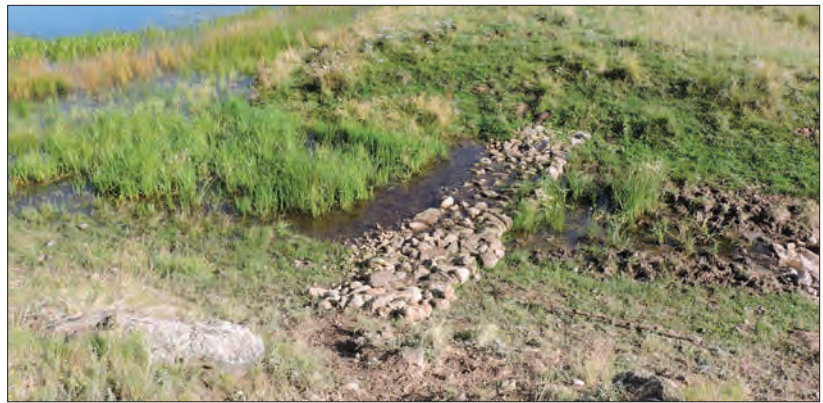
Figure 54. Site 50, August 11, 2015. One rock dam at stock pond outlet. (©W.D. Zeedyk)
