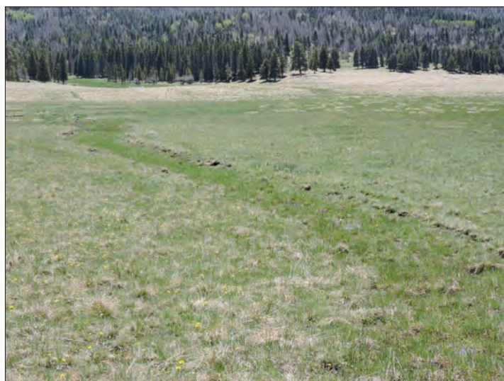
Figure 5. Site 42-44 complex, May 11, 2017. Incision due to cattle trailing in Tributary 3 wet meadow. View looking upvalley. (©W.D. Zeedyk)
