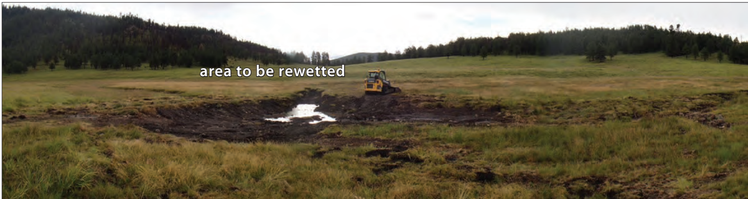
Figure 30. Pond beginning to fill as construction continues. Area to be rewetted is beyond the end of the lead-out channel. (©S. Vrooman)
