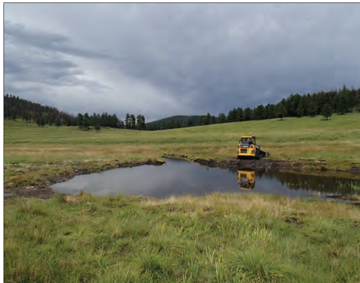
Figure 4. Site 21, August 7, 2016. A plug and pond on a perennial channel fills soon after construction. (©S. Vrooman)
